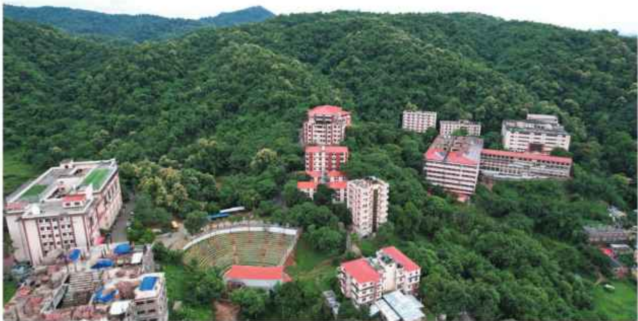
The latest aerial view of the Assam down town University Campus.
